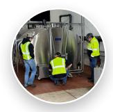
Custom Engineered Tank: Insulated, chilled, agitated, flexible installation depending on needs, a CIP system to meet or exceed USDA dairy standards, as well as all necessary piping to and from the milking parlor.
